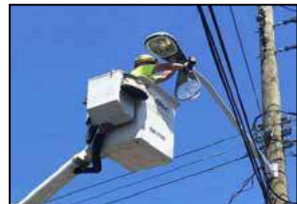
Utility worker retrofitting existing streetlamps with next-generation LEDs
