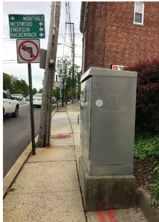
Figure 45: Example of Above Ground Junction Box Interfering with Streetscape in Park Ridge
