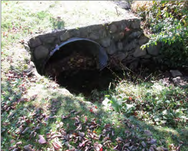
East Allison Avenue Culvert – Example of Stormwater Drainage Infrastructure (Elizabeth Matamoros)
