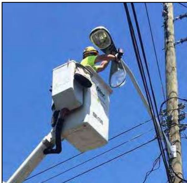
Figure 3 – Utility worker retrofitting existing streetlamps with next-generation LEDs
