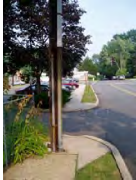
Many sidewalks are in need of repair and modification. In this case, the walkway is interrupted by a utility pole.
